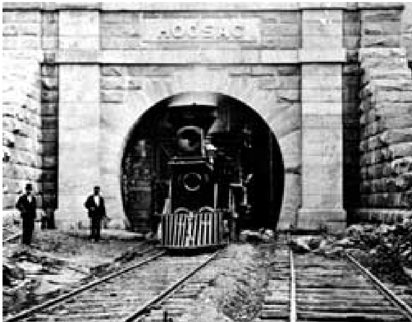
Hoosac Tunnel – West Portal, circa 1875
