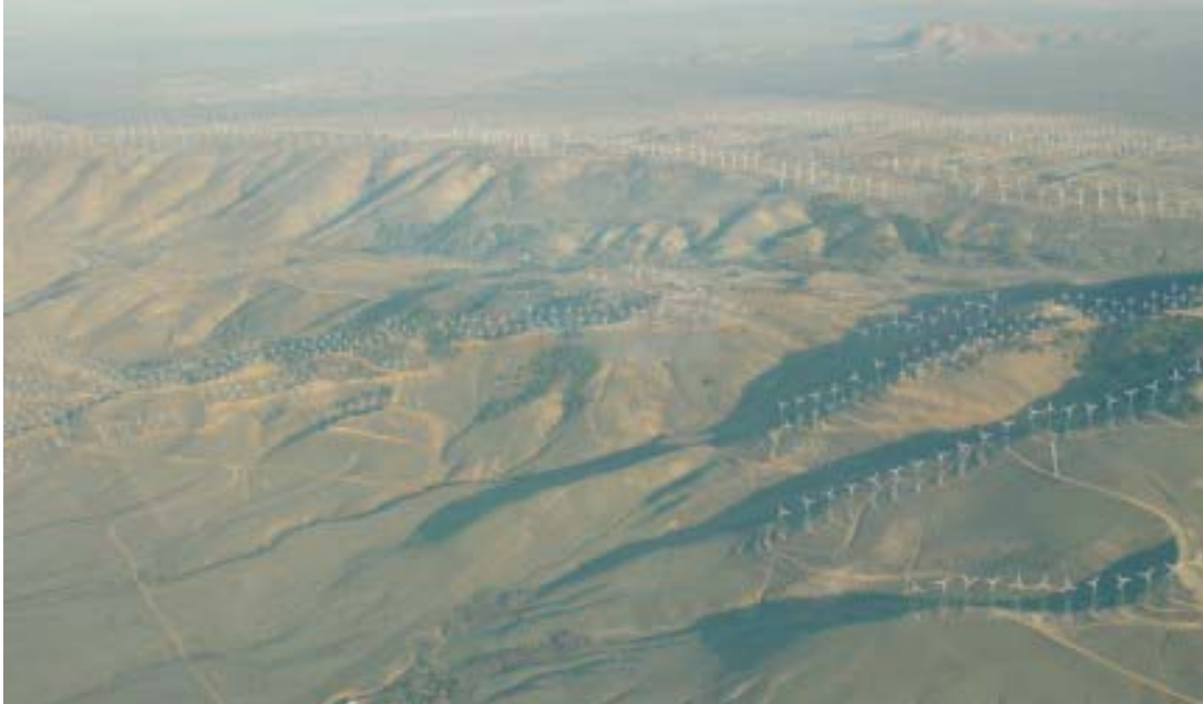
FIGURE 7. TEHACHAPI PASS, TEHACHAPI, CALIFORNIA
