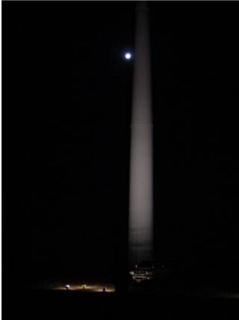
FIGURE 8. EXTERNALLY LIT TURBINE
